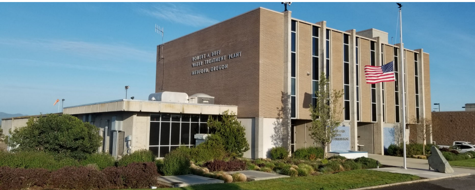
Robert A. Duff Water Treatment Plant
